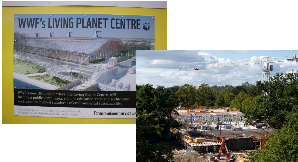
Chantier WWF'S Living Centre Planet
